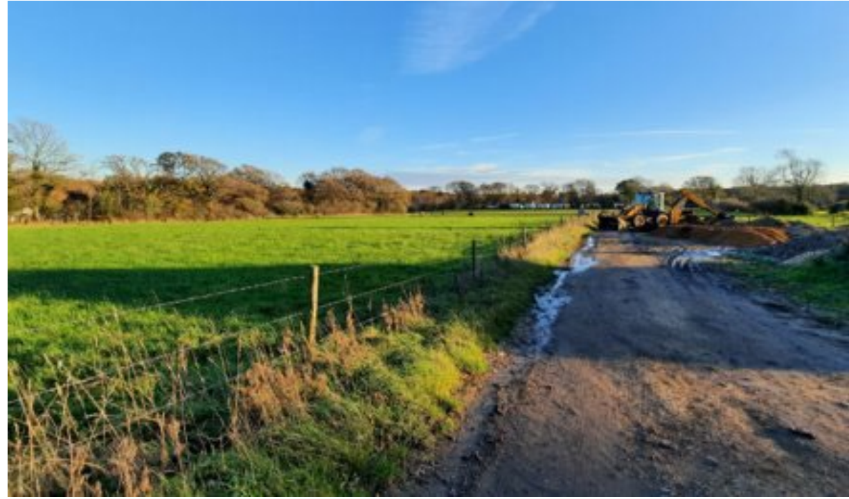
View of site from Sway Road
